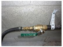
Open the green handled valve inside the generator house, by turning the handle parallel to the pipe as shown in the photo.
