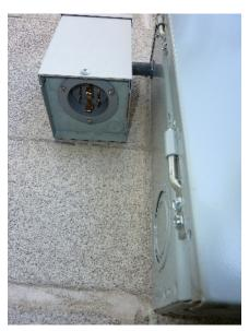
Plug the portable generator into the external outlet to the left of the breaker box using the twist lock cord stored inside.
