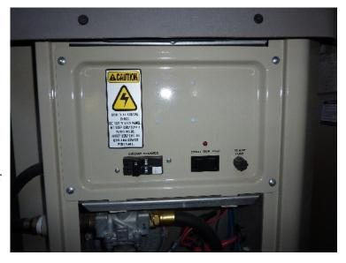
Once the Generator is running check the main transfer switch-breaker panel on the outside wall to make sure the breaker labelled "INSIDE GENERATOR": is in the on position. If not set the switches as shown in the picture below.
