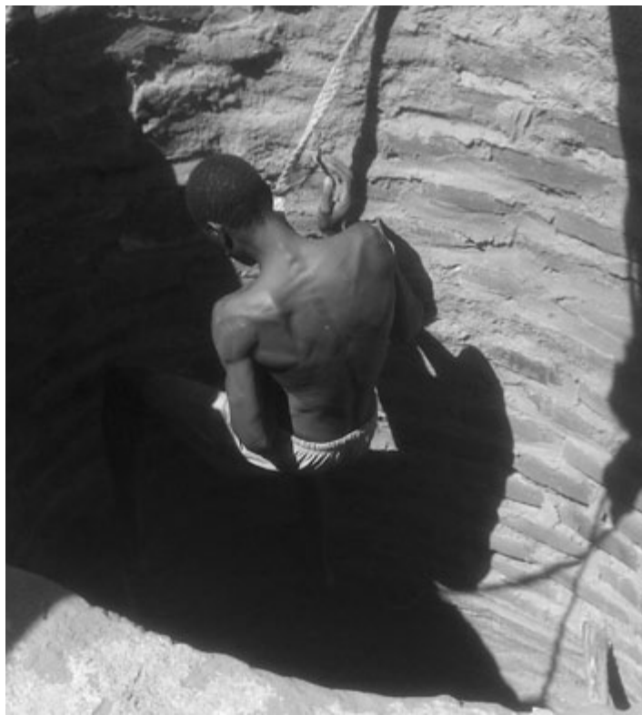
Wambua Kithome lowers himself into opening, where he chips rock and digs a future well.
